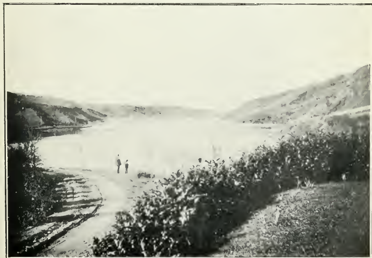
RATHMINES WATERWORKS—THE LOWER RESERVOIR.
