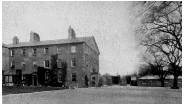
Commandant's House and Entrance Gate
